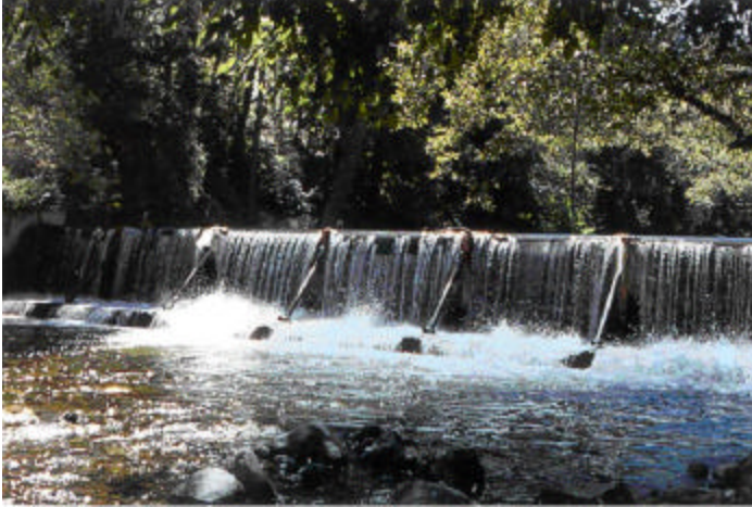
The Buck and Jones Dam on the Little Applegate River.
